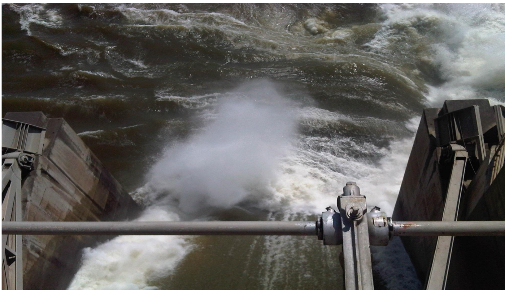
strong cross flow over top of spillbay 15 plunge
