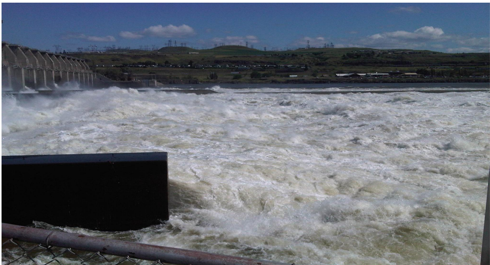
View from north entrance at 200K spill
